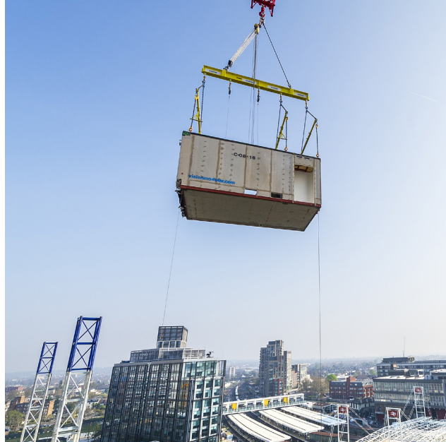
Photo credit: HPA Design, Tide Construction and Vision Modular Systems
